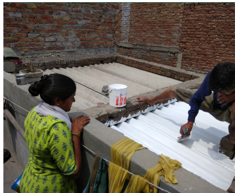
Fig. 2 - Residents of an informal settlement in Bapalal Kadia, Ahmedabad city, India, painting their roof with solar-reflective white paint. [Photo credit: Mahila Housing Trust]
